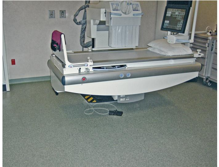
*A poured-in-place urethane mortar system provides this operating room with weldless, long-lasting, stain-resistant floors.*
