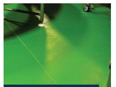
Over 4500 sq. ft. of Stonclad UF was installed with pitch to drains for water flow and drainage.
